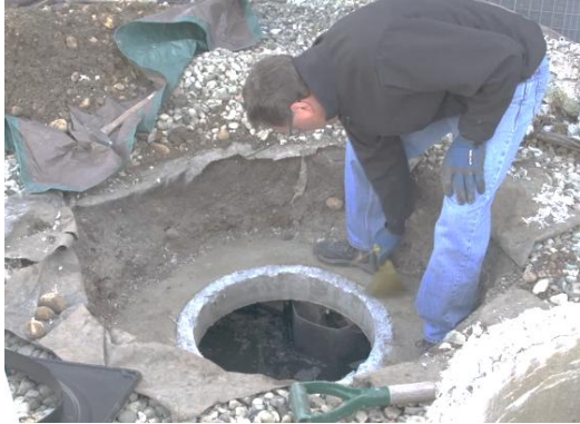
Figure 11: Prepping Tank Surface
